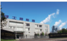
Anhui Lithium Factory
