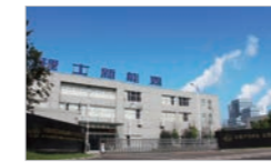
Anhui Lithium Factory
